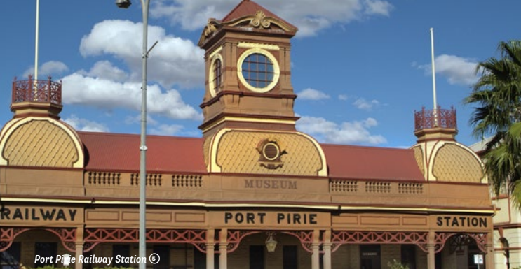
Port Pirie Railway Station ©
